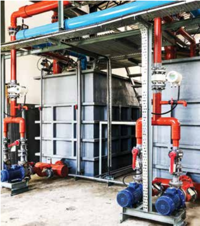
TEK Memplus® with integration of membrane filtration in POME tertiary treatment.
