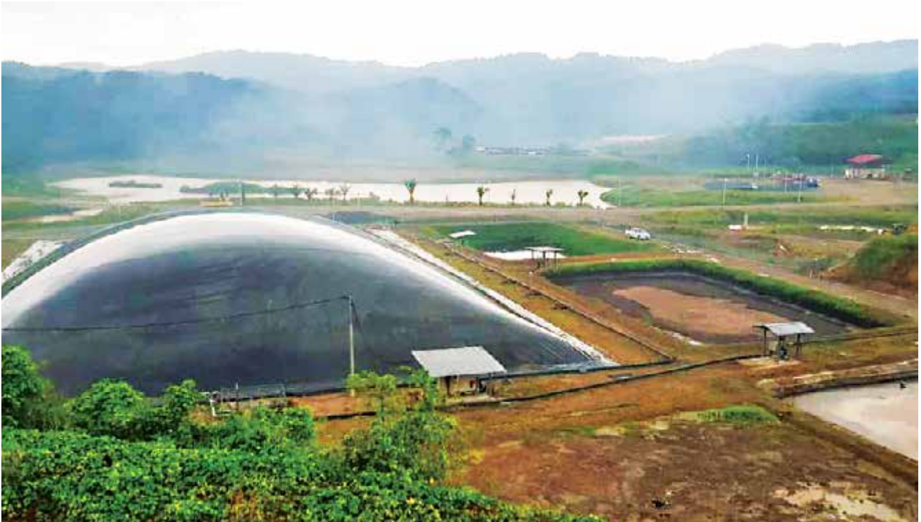
TEK - completed project for biogas (MCLplus®) with improved POME management system.
