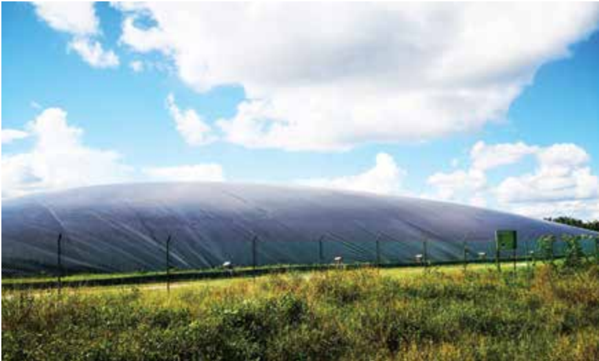
TEK - modified covered lagoon (MCLplus®) for biogas capturing system.
