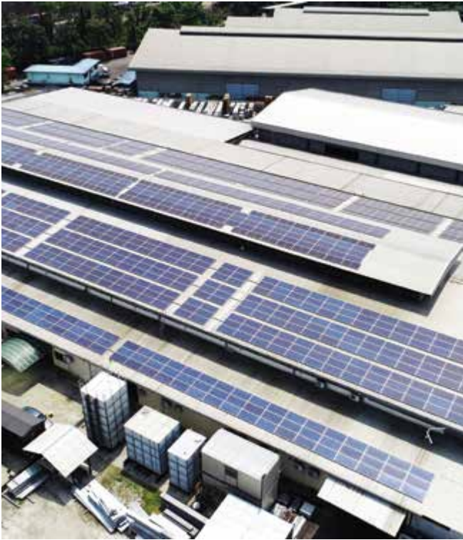
Tera - installed 332kw p Solar Photovoltaic (PV) in Klang.
